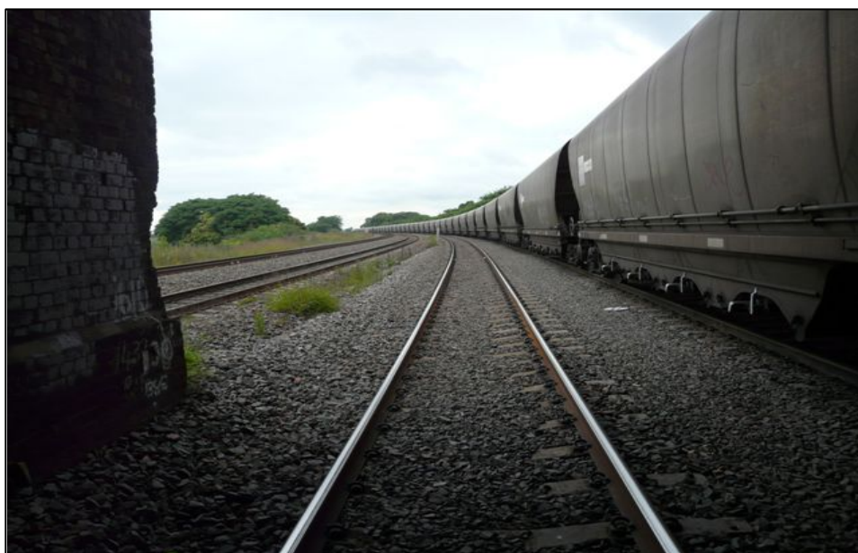
Figure 6: Visibility from the worksite, beneath High Street Bridge
